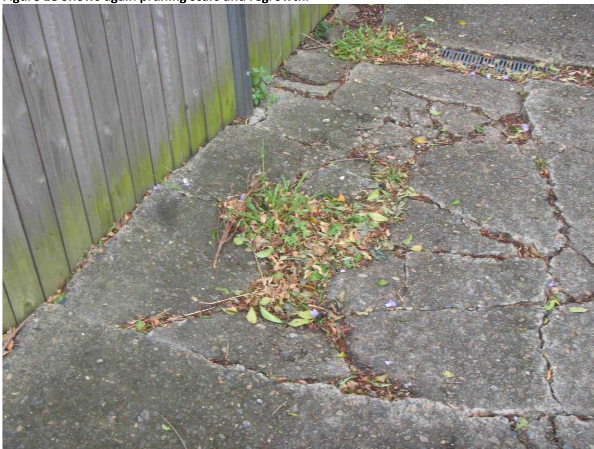
Figure 19 Shows damaged and lifted concrete within the adjoining unit driveway from Tree 7.
